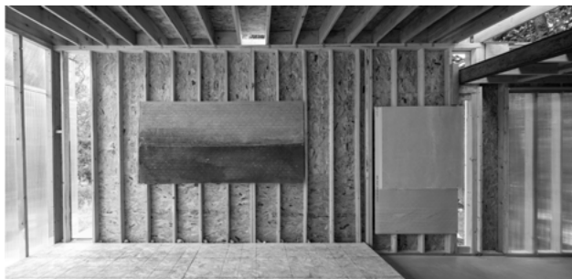
From A Morning in Little Italy , Photo: © Dan Schwalm
